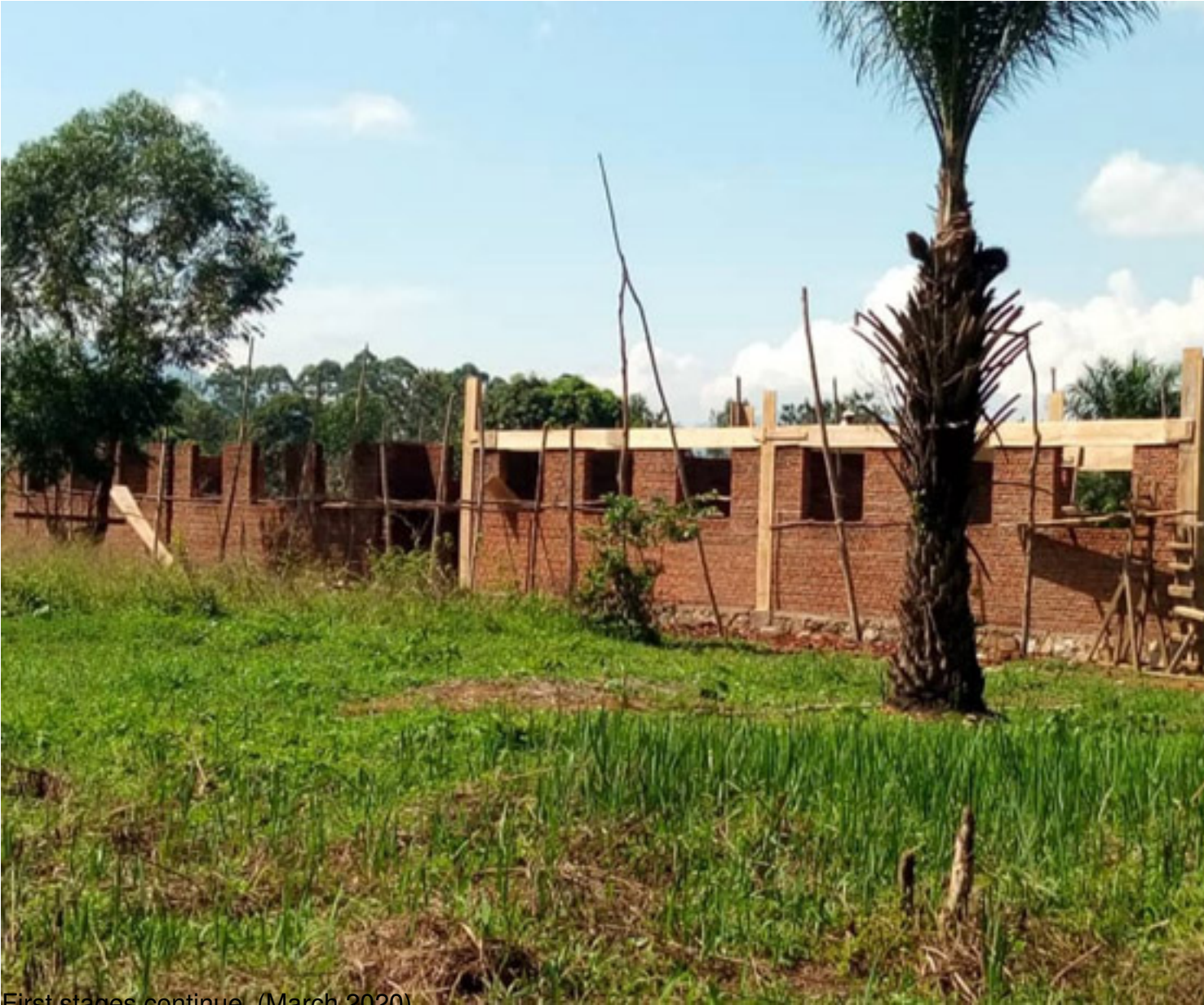
First stages continue (March 2020)
