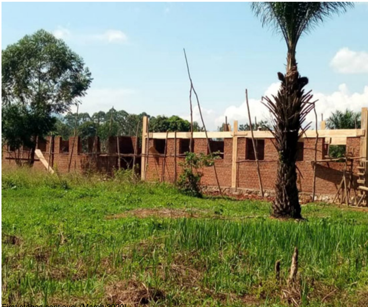
First stages continue (March 2020)
