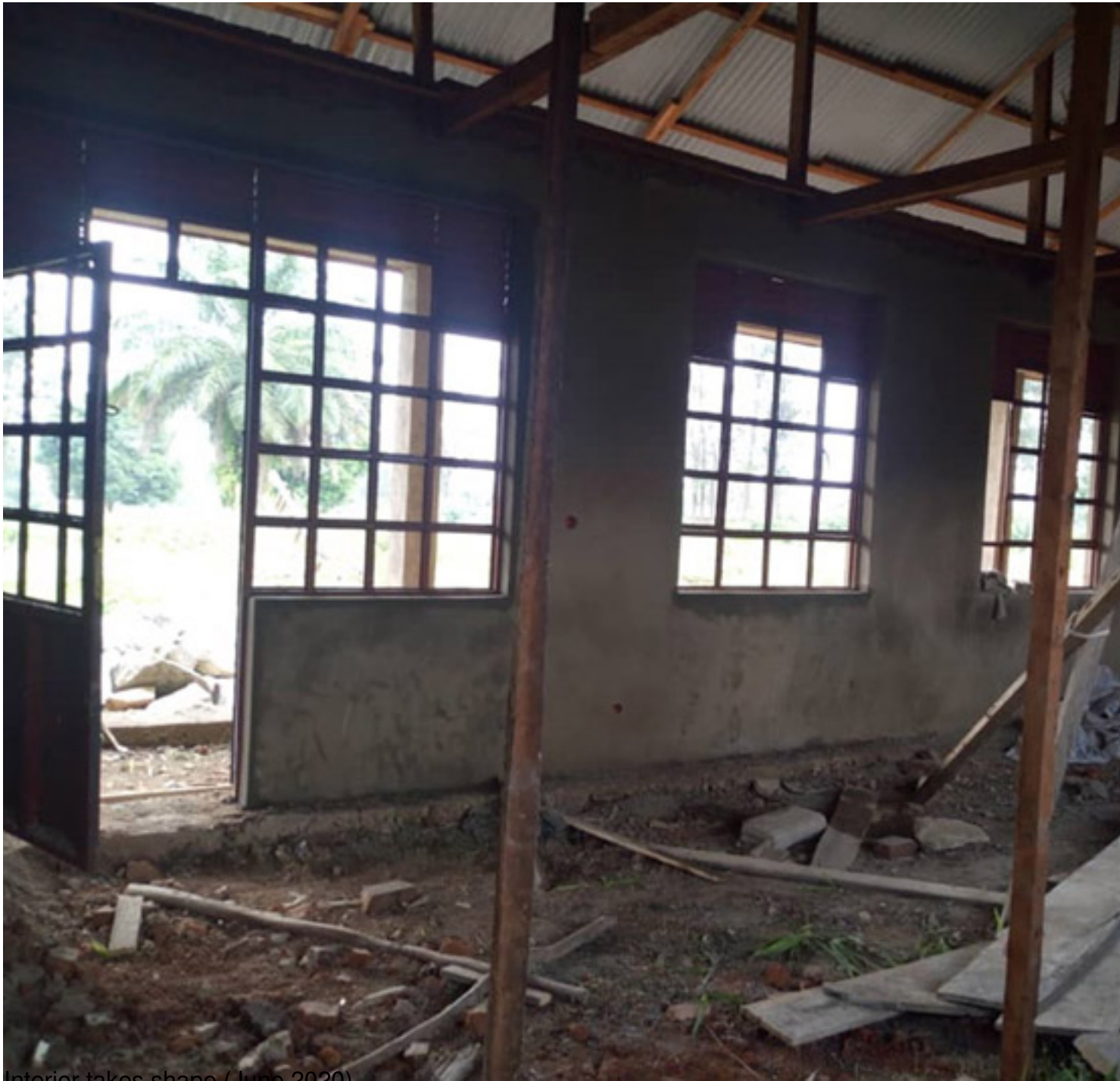
Interior takes shape (June 2020)
