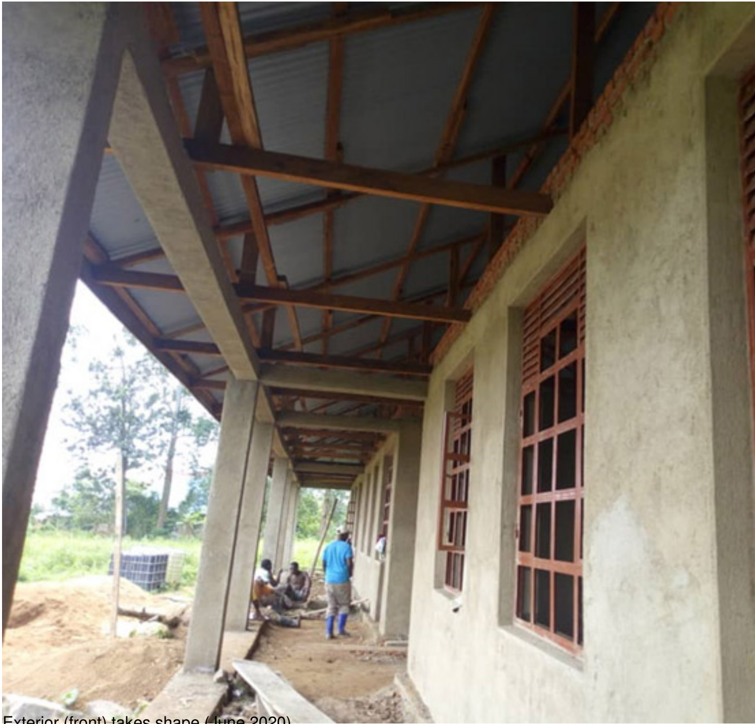
Exterior (front) takes shape (June 2020)
