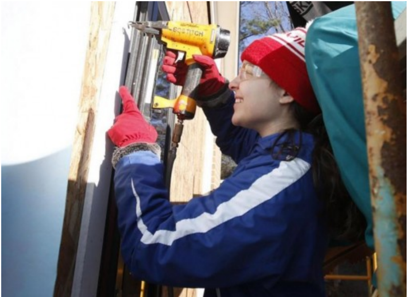
Assumption College students repair homes in Tuscaloosa
